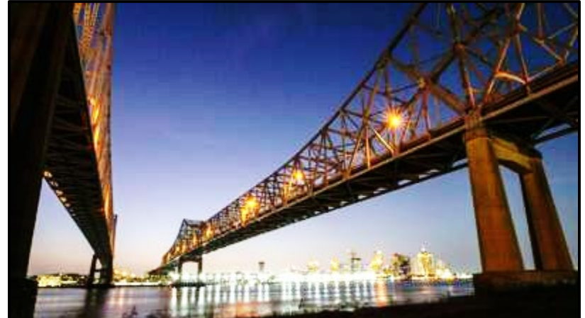
The original lighting system is being replaced by a new LED system.
